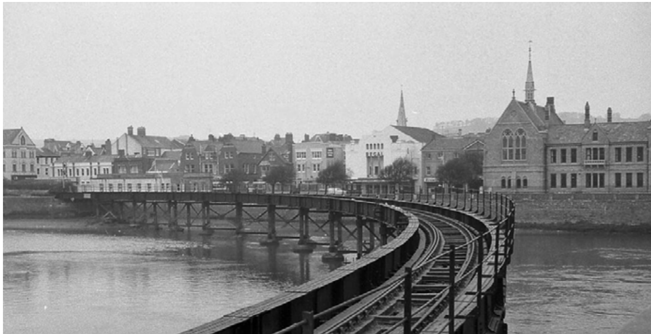
Photograph 3 : Railway bridge over River Taw (Barnstaplehistory.com)
