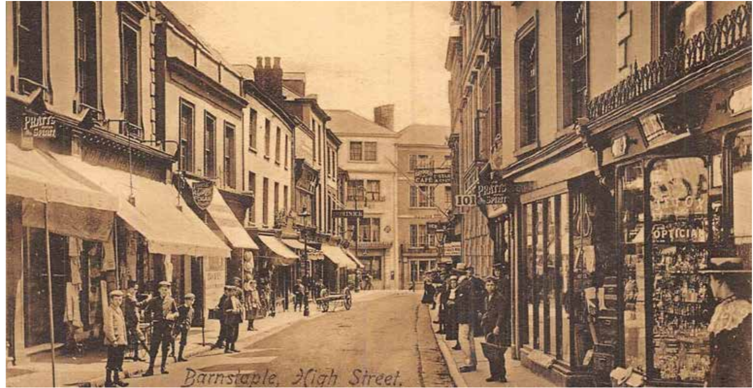
Photograph 2 : Barnstaple High Street (Barnstaplehistory.com)
